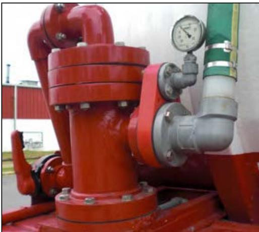
Machined port allows for access to product line
